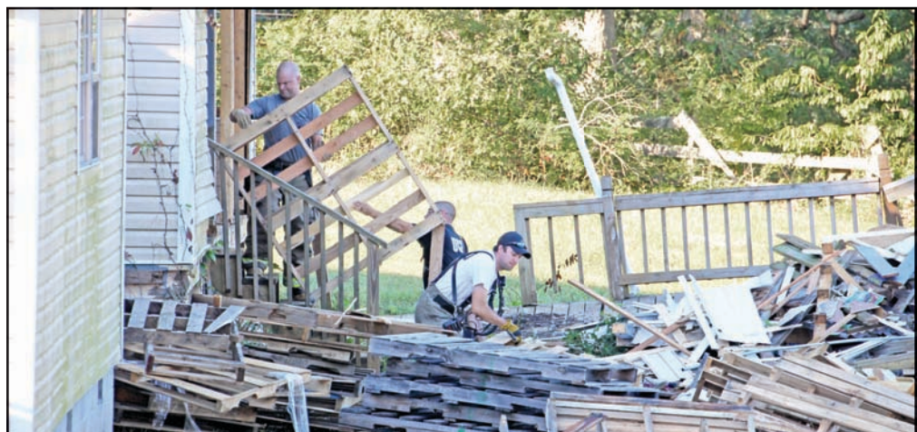
Wooden pallets were used to simulate furniture that had caught fire inside the building.
